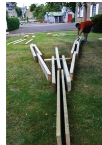
Assembling the Tower
