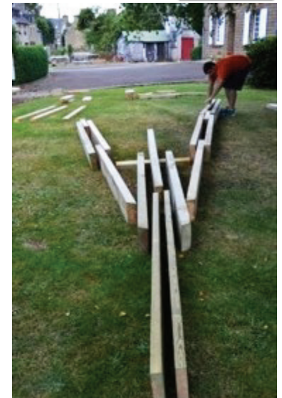
Assembling the Tower
